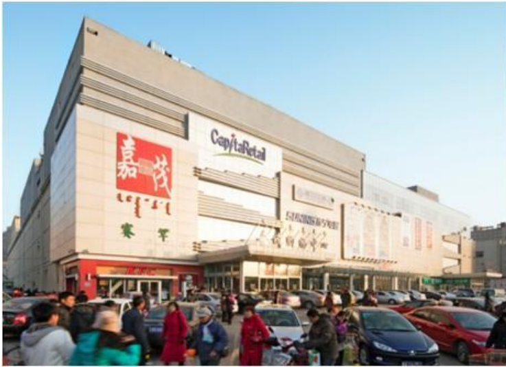
New façade of Saihan Mall
